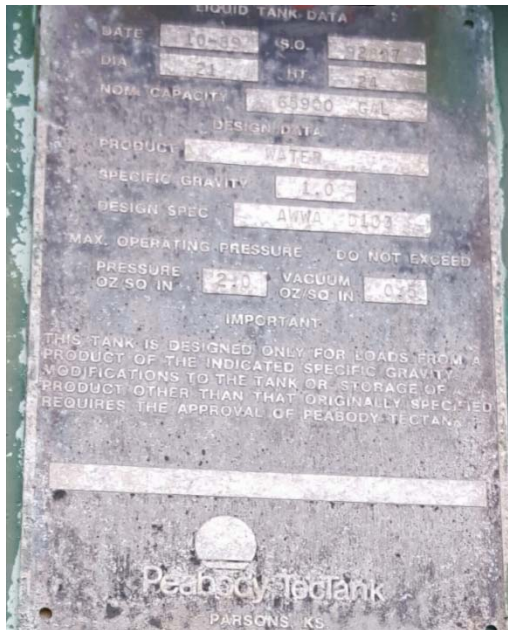
Existing Olosega Tank Information Plate.
